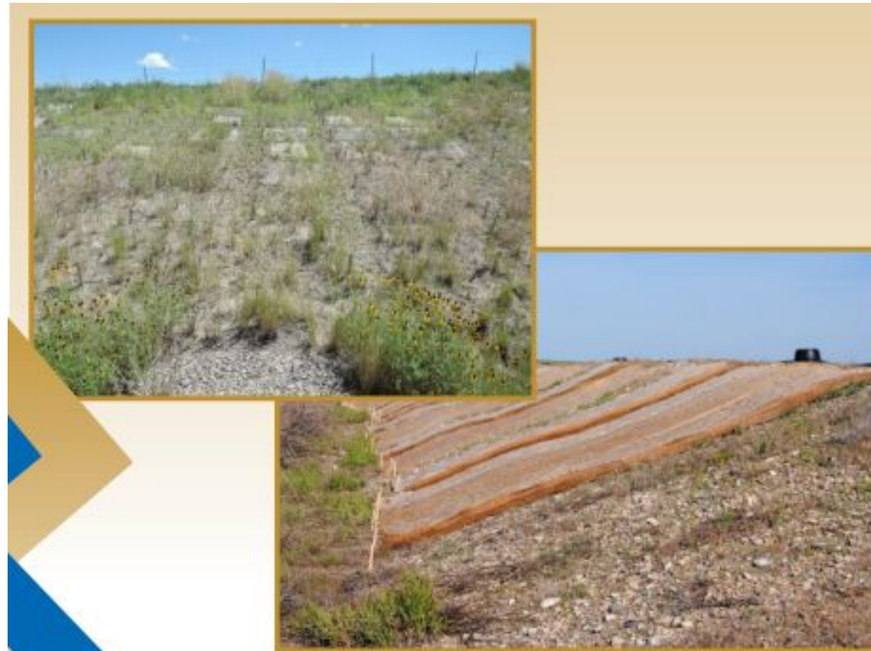
Figure 7: Demonstration of two erosion control blankets using different ratios of wool and straw produced by Ero-Guard.
