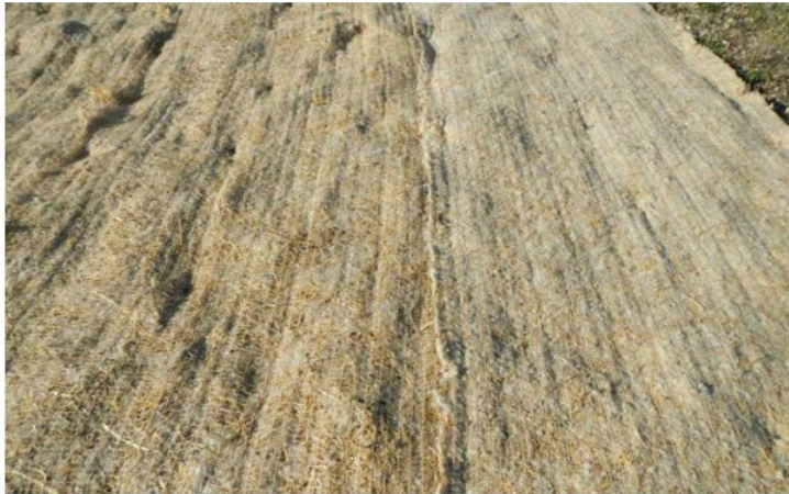
Figure 7: Demonstration of two erosion control blankets using different ratios of wool and straw produced by Ero-Guard.
